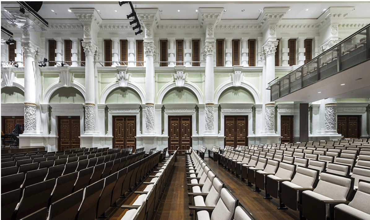
THEATRE BALCONY RAILINGS AT VICTORIA THEATRE
