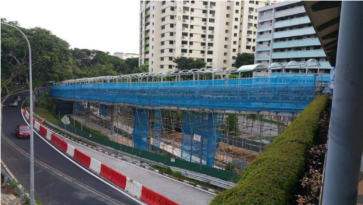
OVERHEAD LINKWAY AT C928 BEDOK TOWN PARK STATION
