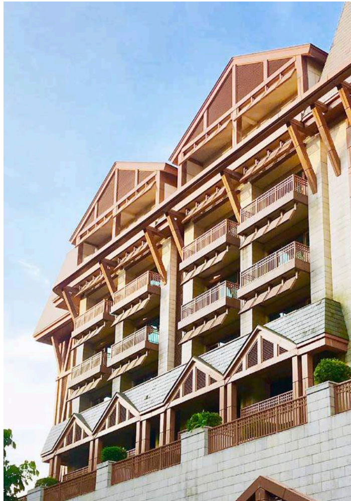
RAILING FACADE AT EQUARIUS HOTEL @ RESORTS WORLD SENTOSA
