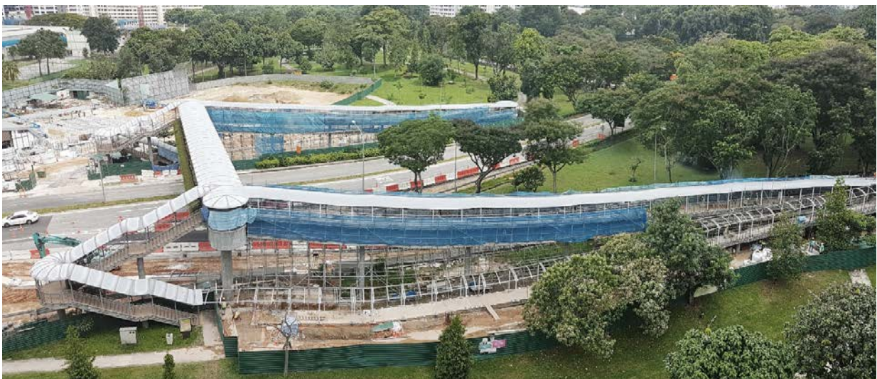
OVERHEAD LINKWAY AT C928 BEDOK TOWN PARK STATION
